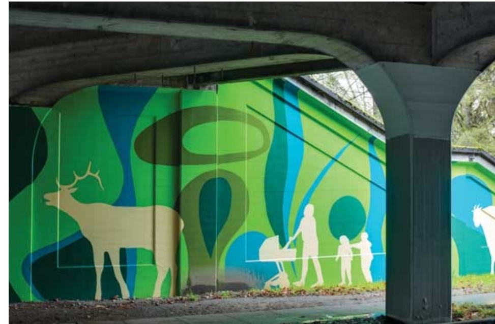
Bridge Underpass, Seattle
